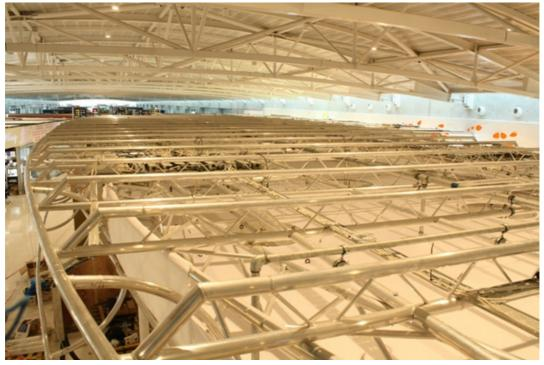
An oval structure permanently sited indoors, created in two independent sections either side of an "earthquake-proof" movement joint. A grid of aluminium truss tubes carrying internally lit fabric, LCD projectors and services, cantilevers over the edge of two semi-elliptical rings of lattice truss supported off a combination of hollow section aluminium tubes and truss legs. Fabric covered lamps hang beneath the semi-elliptical rings.
